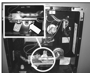
Water Heater Drain Plug Location
