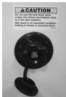
Tank Flush Inlet
